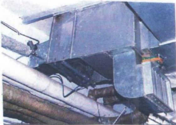
Mdoifield AHU with fresh air fans
