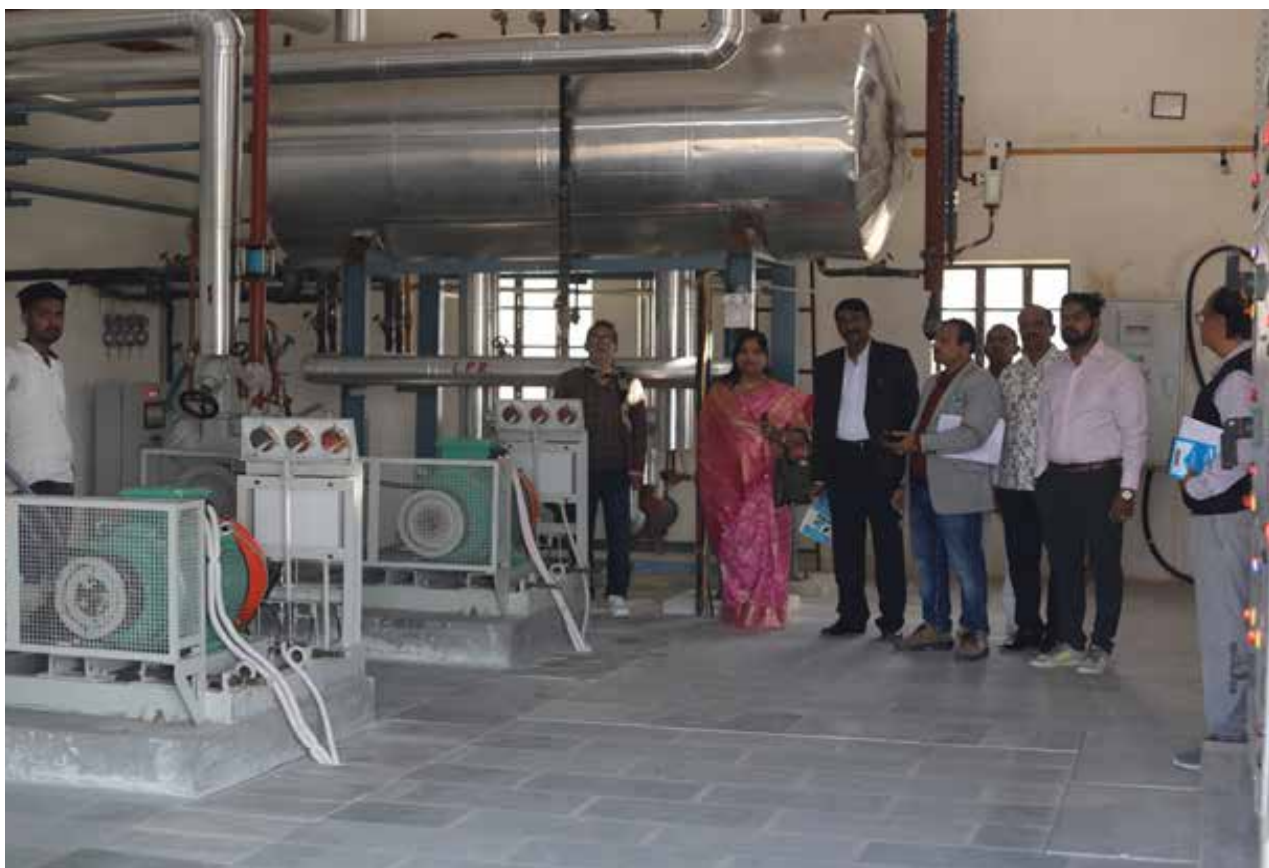
NHB assisted Cold Storage project at Telangana
