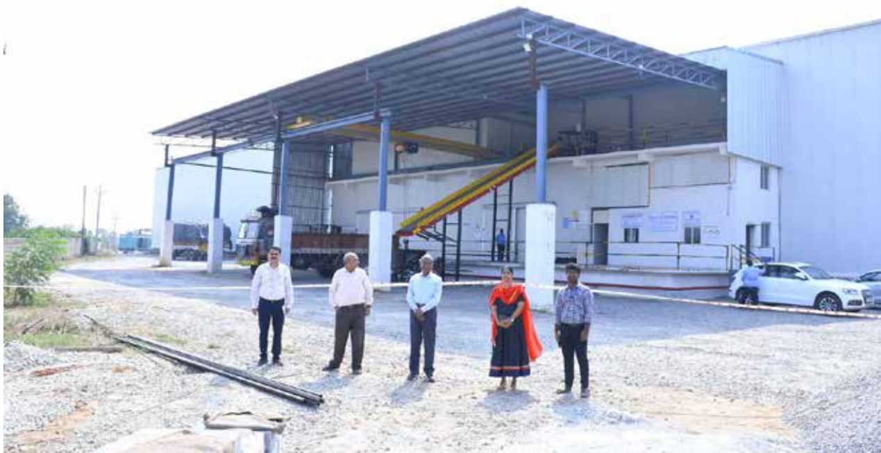
NHB assisted Cold Storage project at Telangana
